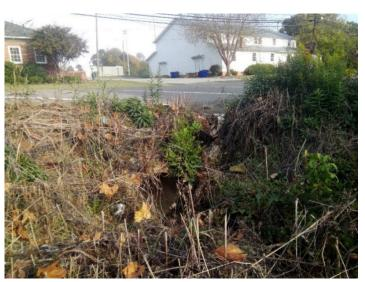
Figure 14: Clogged/Broken Outfall Pipe and Litter on Third Ave.
