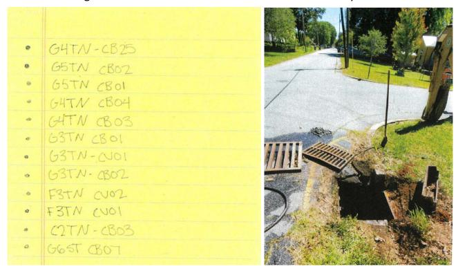
Figure 10: Catch Basin Full of Sediment (Cleaned 5/2020)
