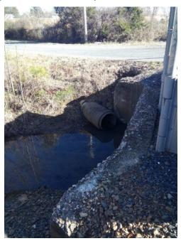
Figure 16: Outfall Pipe with Oil Sheen
