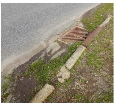
Figure 12: Erosion of Curb Next to Catch Basin on West Raleigh Street
