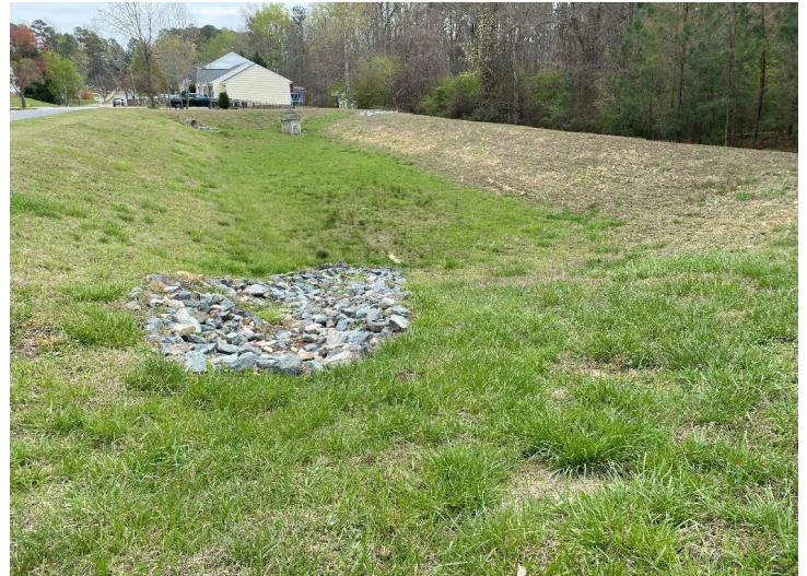
Figure 46: Existing Dry Detention Basin by Holly Springs Police Station,, to Retrofit to Stormwater Wetland
